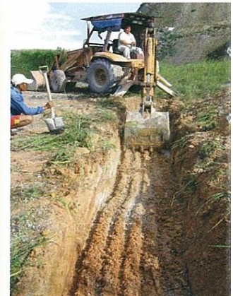
Trench excavating
