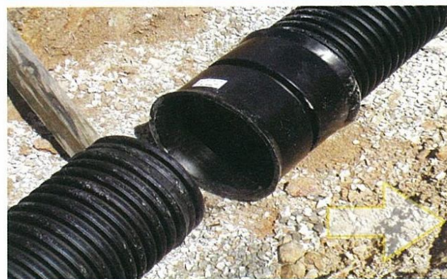
Align the next pipe with the socket and repeat Step 1 and 2
