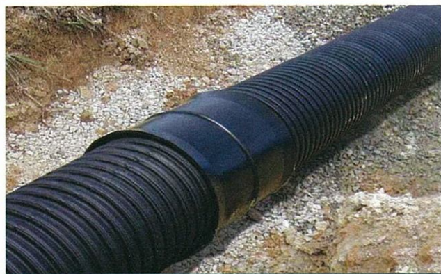
Push socket into pipe carefully, ensuring that the socket ends are protected from damage
