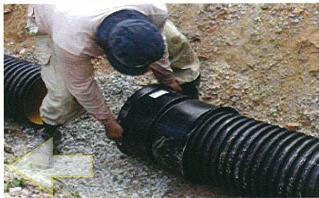
Align and insert socket into pipe
