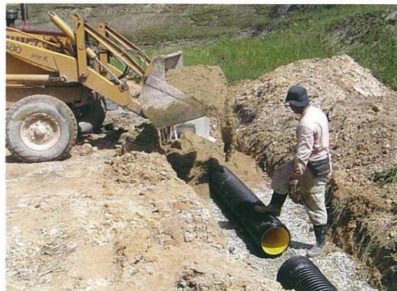
Backfilling of sewer pipe
