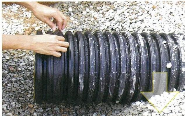
Insert rubber ring onto the second valley of the pipe
