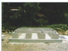
Base Concrete PAD
